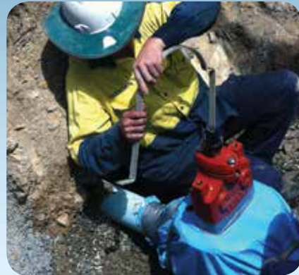
An InsertValve installation under full line pressure.
