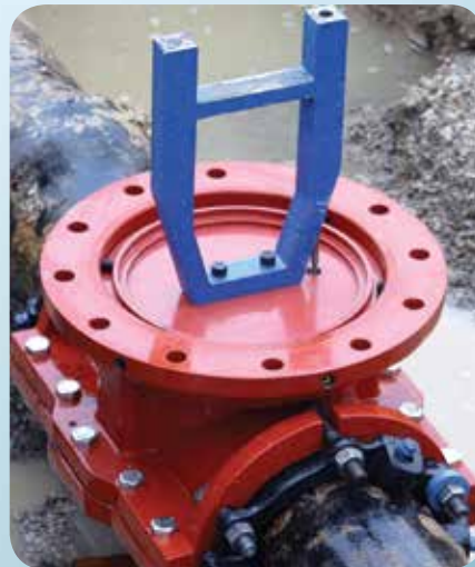
Internal equalization completion plug installed.
